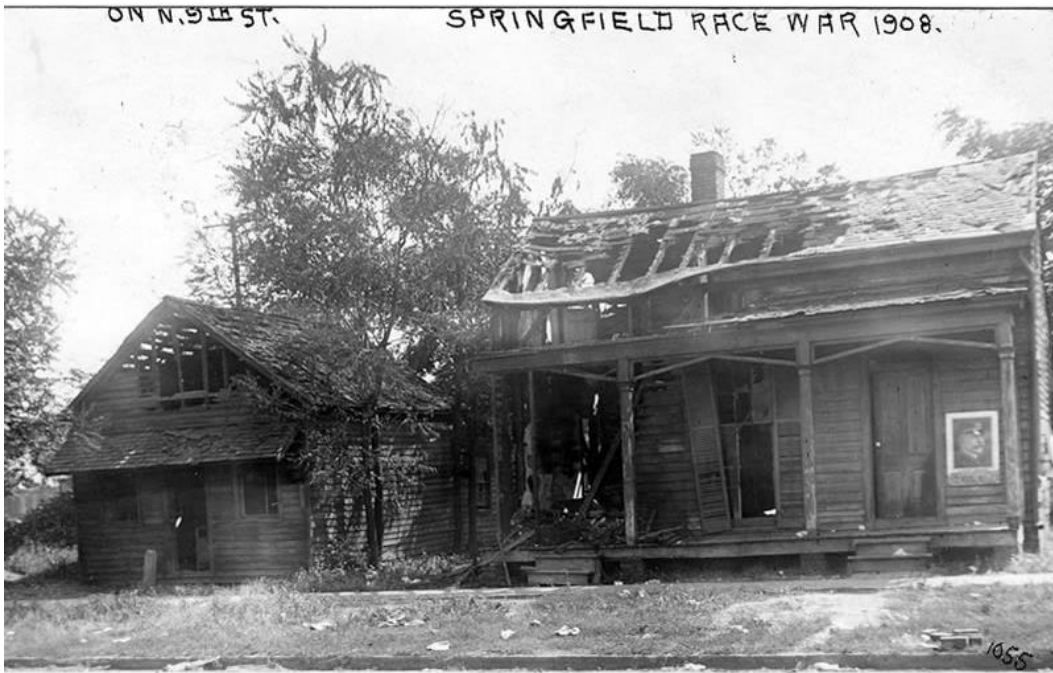
View 4b. Burned-out houses at 312 and 314 North Ninth Street, looking east (ALPLM Ide Collection PC11a; Sangamon Valley Collection 90-387A008).
