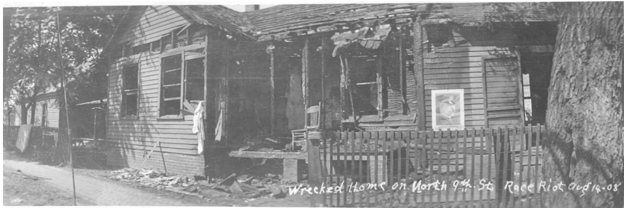
View 3a. Wrecked houses on the west side of the 300 block of North Ninth Street, looking southwest (ALPLM Ide Collection NG5798).
