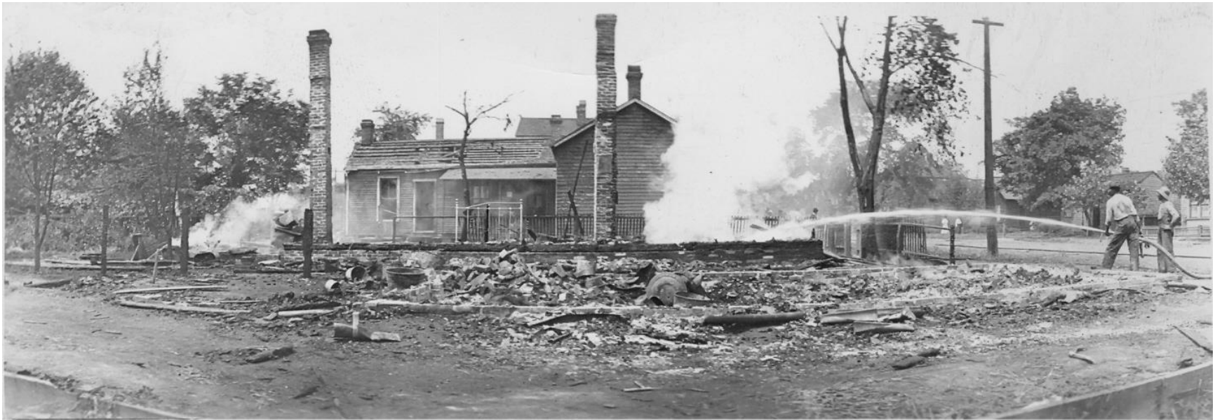
View 17a. South side of the 1100 block of East Mason Street, looking west and showing ruins of houses at numbers 1128 and 1130 in foreground and damaged house at 1126 in background. Top: From 1909 scrapbook (Smithsonian African American History Museum). Bottom: ALPLM Ide Collection, NG5793. Two of the occupants of these homes were William Brandon, a barber, and James Caldwell, a shoemaker, both of whom were Black.
