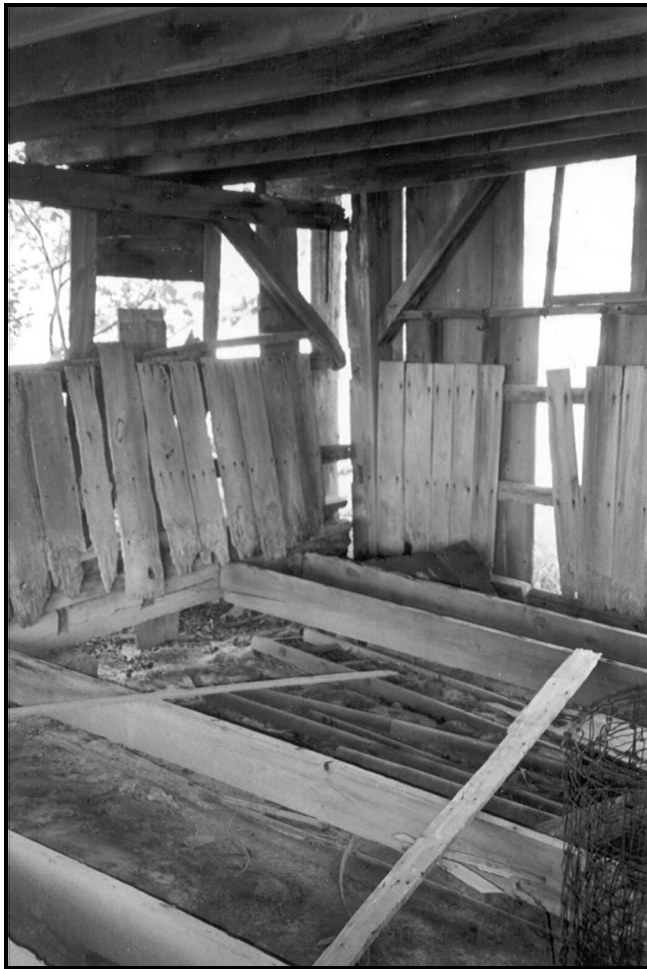
Figure 10. (LEFT) Interior view of the eastern box stall in the north bay of the barn. The vertical planking nailed around the lower part of the walls served as a rub guard, protecting the main framing and exterior siding from wear or damage by livestock. The flooring in this part of the barn also has been removed, as have many of the joists. (RIGHT) View of one of the grain bins located in the south bay of the barn. The ceiling and wall adjacent to the central drive was left open in order allow grain to be tossed into the bins. Tight siding used to enclose the grain bins is indicative of small-grain storage, in contrast to the spaced-out slats typical of corncribs. (FRR October 2002).
