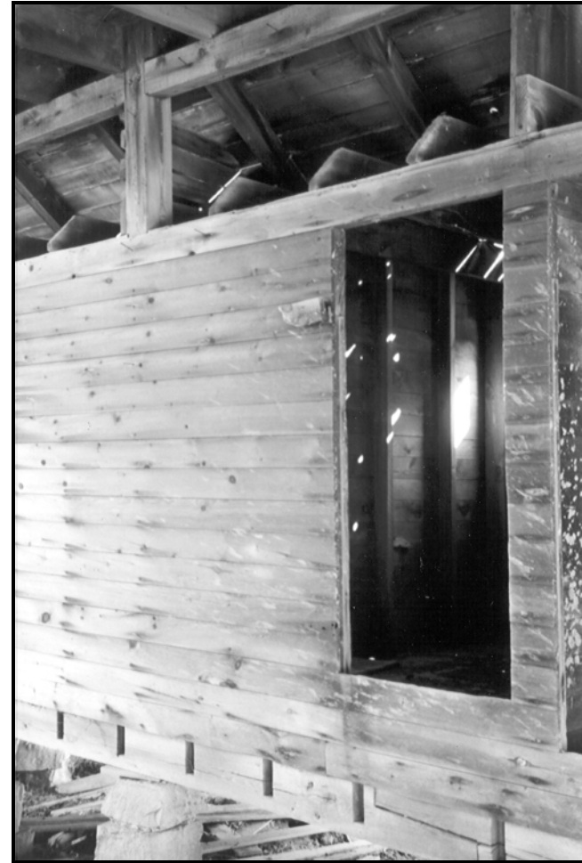
Figure 10. (LEFT) Interior view of the eastern box stall in the north bay of the barn. The vertical planking nailed around the lower part of the walls served as a rub guard, protecting the main framing and exterior siding from wear or damage by livestock. The flooring in this part of the barn also has been removed, as have many of the joists. (RIGHT) View of one of the grain bins located in the south bay of the barn. The ceiling and wall adjacent to the central drive was left open in order allow grain to be tossed into the bins. Tight siding used to enclose the grain bins is indicative of small-grain storage, in contrast to the spaced-out slats typical of corncribs. (FRR October 2002).
