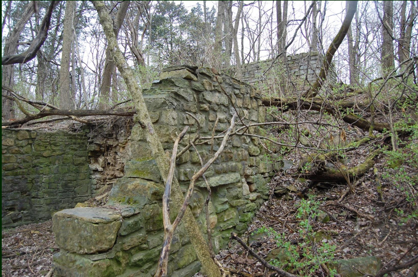
View looking uphill from cellar floor level to level of Wine House floor.
