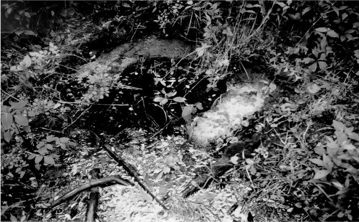
**Figure 3. Photograph of the springhead, looking north (2000). The upper part of the concrete shaft surrounding the springhead has deteriorated on its south side.**
